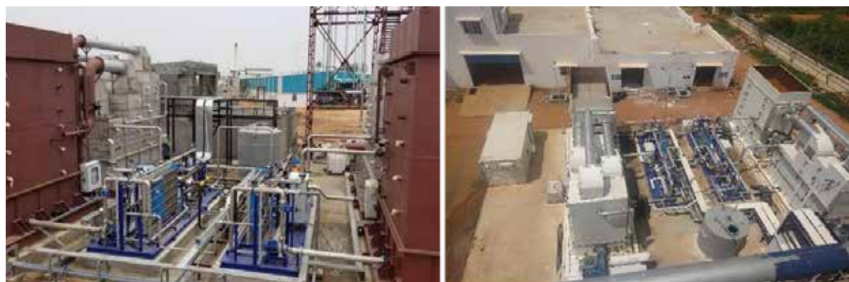
Figure 1 A typical CGE system at an Indian textile processing mill - Humidifier & De-humidifier columns along with pump skids
